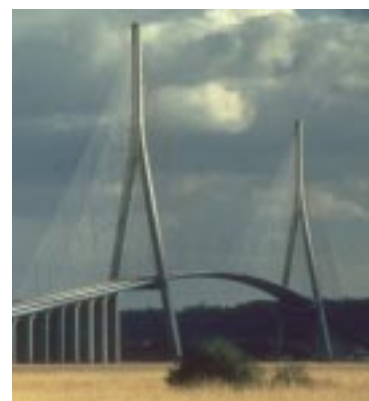
The Normandie Bridge, the longest span cable stayed bridge in the world with a main span of 856m.
