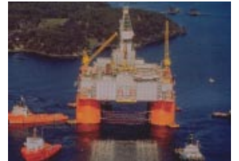
The Snorre Development Project Norway. This tension leg offshore platform is anchored at depth of 310m. It is the longest of its kind in the world.
